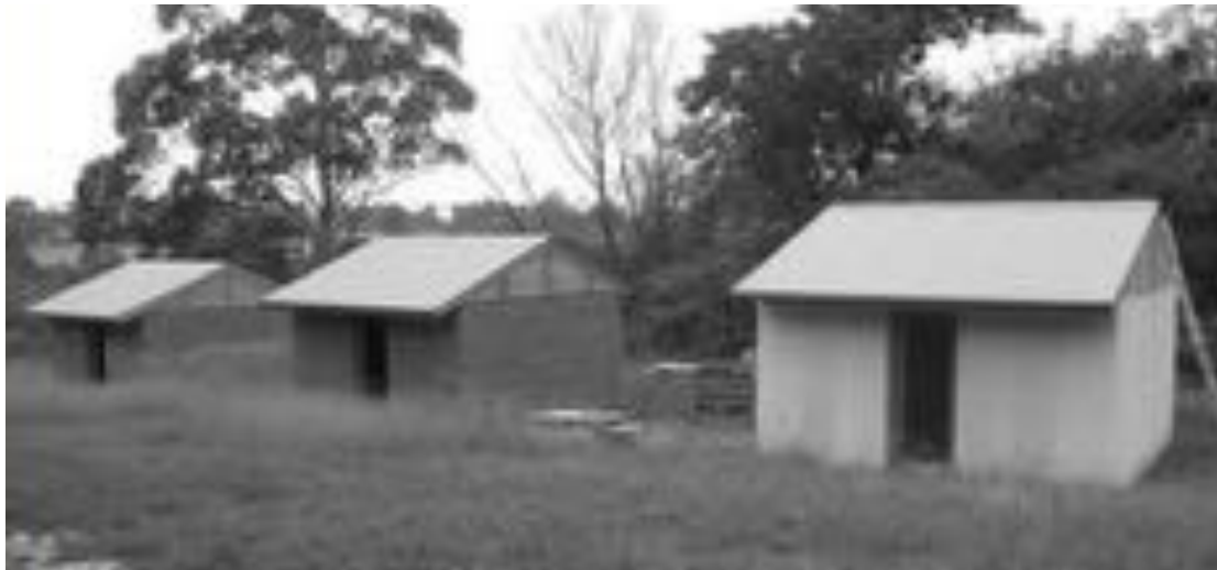
Figure A1.22 – UTS Test Buildings Photograph
