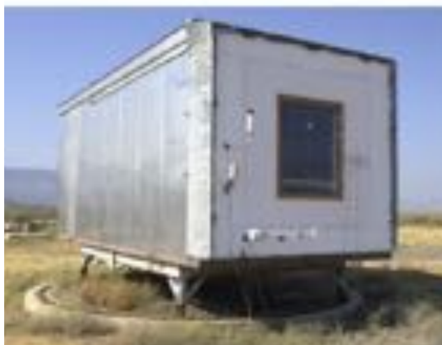
Figure A1.18 – PASSYS/PASLINK Test Building Photograph
