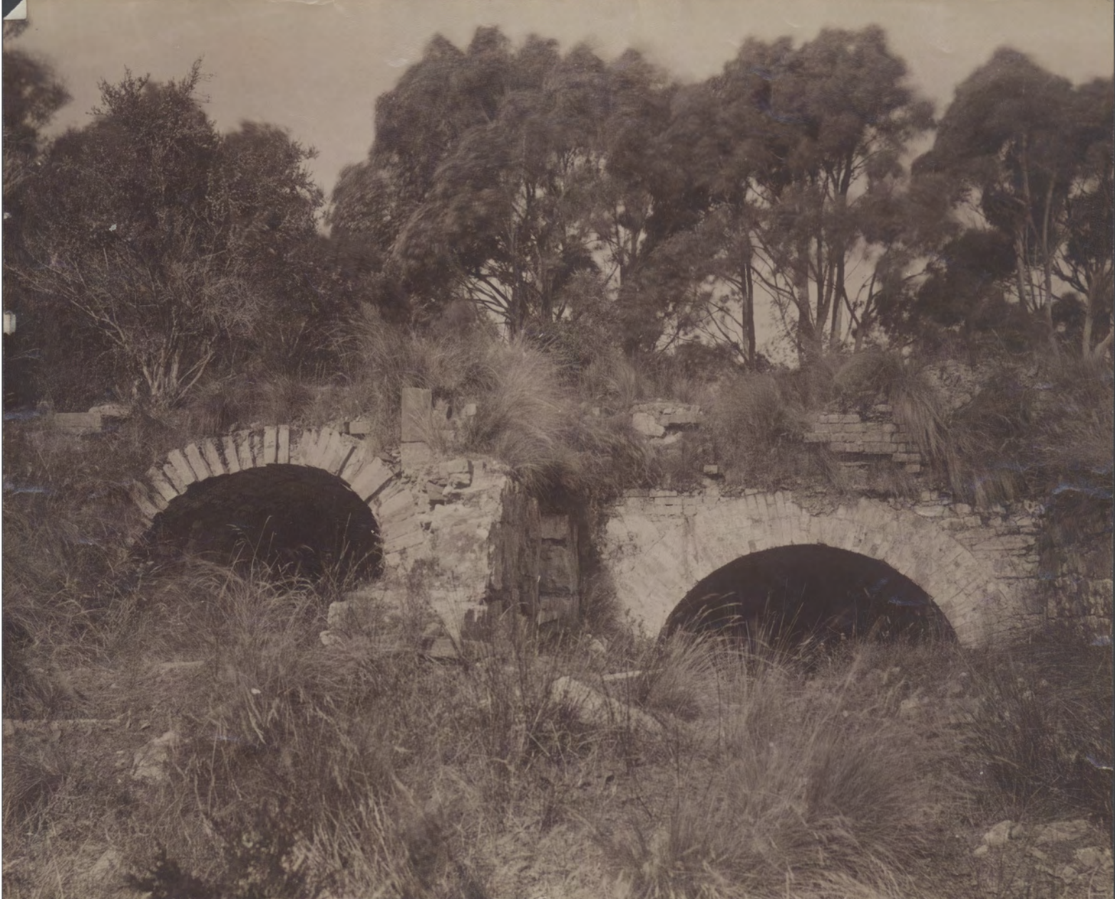
UNDERGROUND CELLS, POINT PUER, PORT ARTHUR, ANSON, HOBART, 310B
