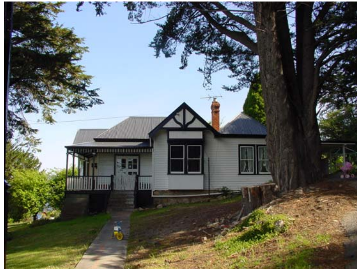
Figure 1. Taroona house subject to retrofit (Weaver, 2005, p.86)
