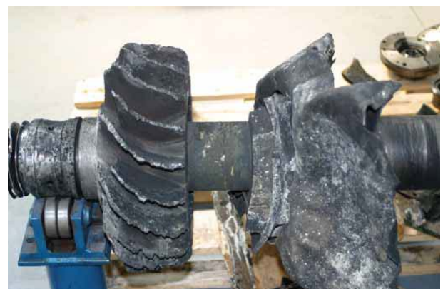
Figure 9. Damaged turbocharer rotor shaft ( Courtesy : ATSB Investigation 186 and 191)
