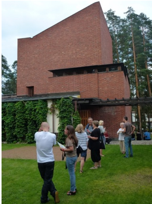
Figure 4.6 AALTO SÄYNÄTSÄLO Town Hall, council chamber Photograph by John Roberts, 2011
