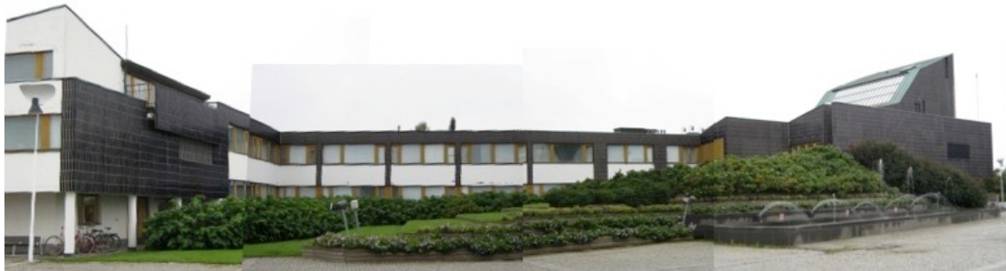
Figure 4.21 AALTO Seinäjoki Town Hall Photograph by John Roberts, 2008
