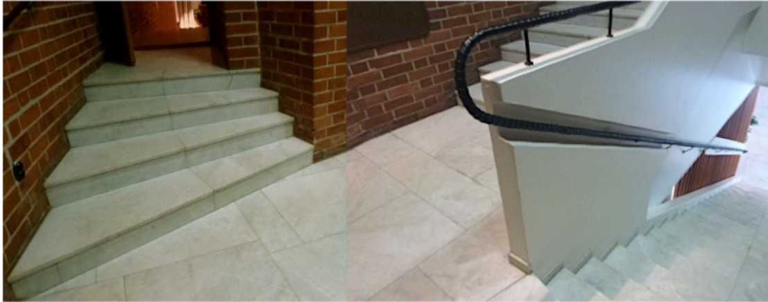
Figure 3.31 AALTO Jyväskylä Festival Hall, stair landing Photograph by John Roberts, 2008
