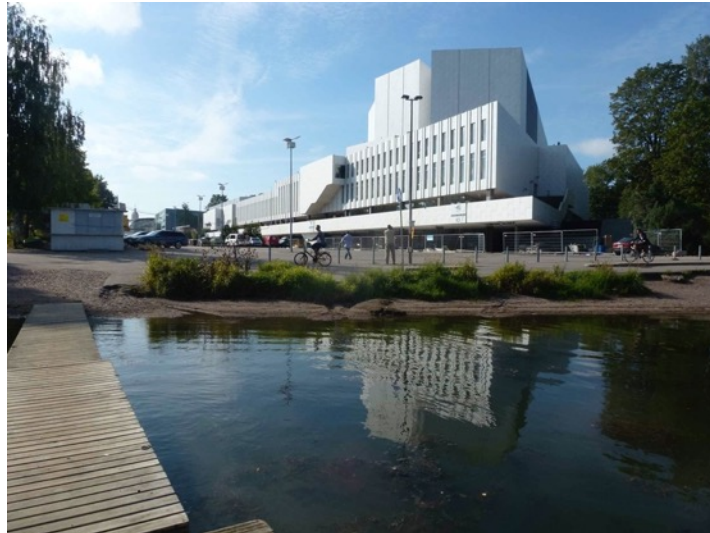
Figure 4.32 AALTO Finlandia Hall Photograph by John Roberts, 2011
